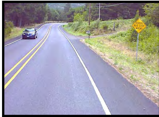
LONDON ROAD AT MP 1.69
