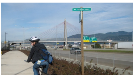
Grade-separated crossing over I-5
