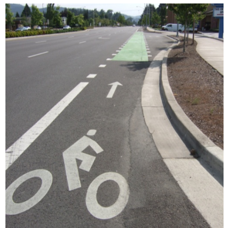
Bike lane next to the car travel lanes, includes green paint where cars turn into a parking lot
